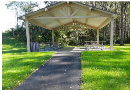
New Shelter replaced burned shelter
